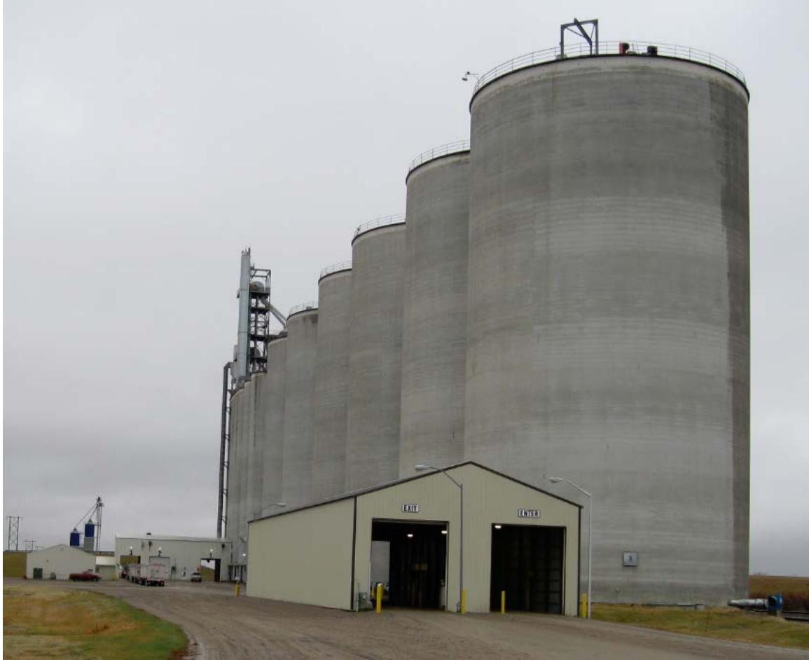
Image 2. Alton Grain Terminal, truck weighing and dumping; 3 dump pits with 45 trucks/hour capacity
